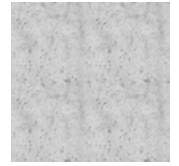
Masonry Concrete Splintered QP28
