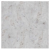
Masonry Concrete Stained QP29
